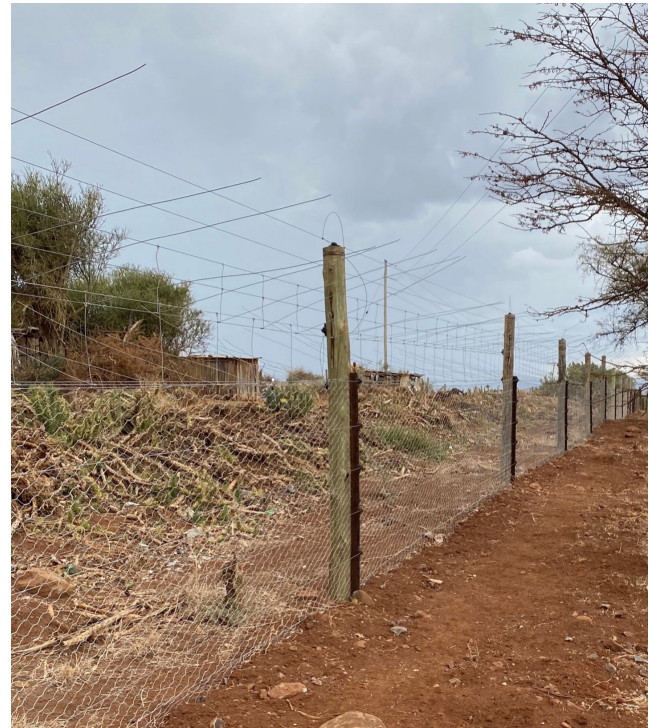
FIGURE 2 Newer design predator-proof fence with buried mesh, electrified butterfly outrigger stingers and electrified posts. (Photo M. Dupuis-Desormeaux).
