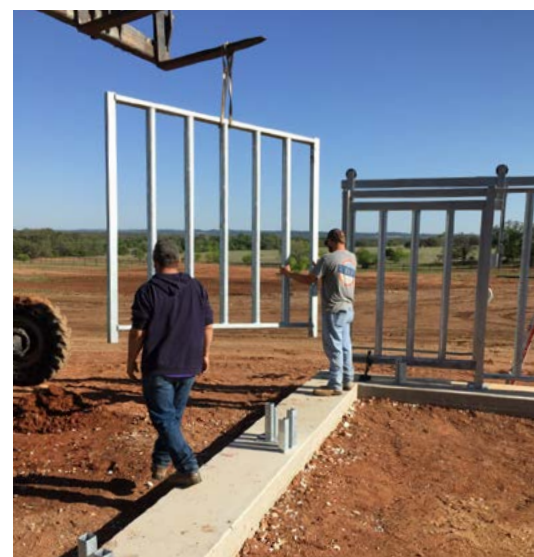
Installing rhino containment panels and gates.
