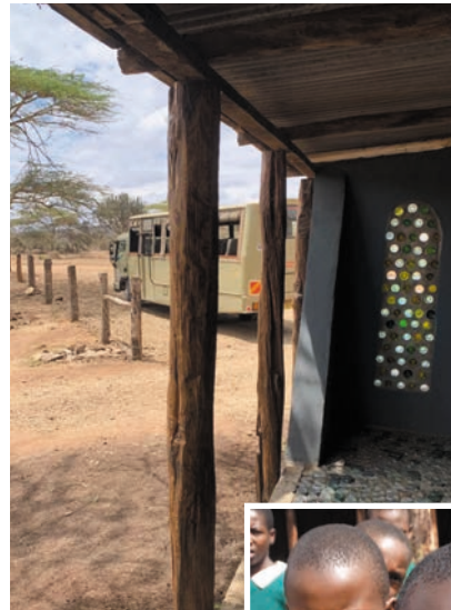
Left: The Mazingira Yetu building has been built sustainably using local and recycled material from in and around Borana Conservancy.
