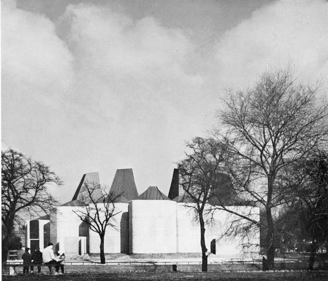
58. The new Elephant and Rhinoceros Pavilion at London Zoo provides a visual parallel to a group of elephants at a water-hole (see pp. 123-25). The building is roughly circular in shape and on each side there is a large, semi-circular animal enclosure containing trees and ponds. The moats separating the animals from the public follow roughly the same curve as the rounded walls of the building itself. The tall roof hoods that dominate the exterior are placed over the animal dens and light them from above. Henk Snoek/Casson Condon & Partners
