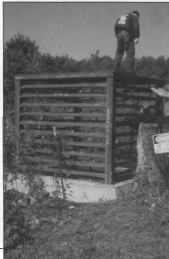
Cage over vertical air shaft being inspected.
