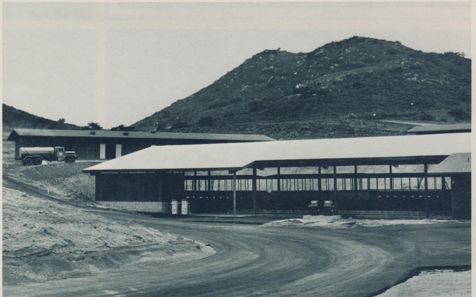
The "car barn" for 19 monorail cars (18 passenger, 1 flatbed).
