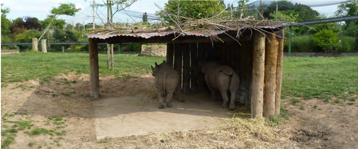
Figure 2.7: An outdoor rain / sun shelter
