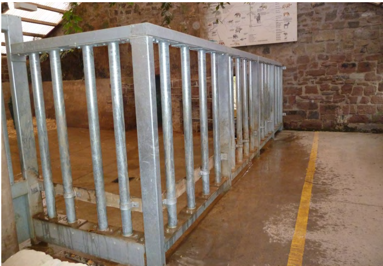
Figure 2: Indoor barrier between rhinos and keepers that allows keepers close contact to the rhinos. Note the low horizontal barrier that prevents a young calf passing through the bars.
