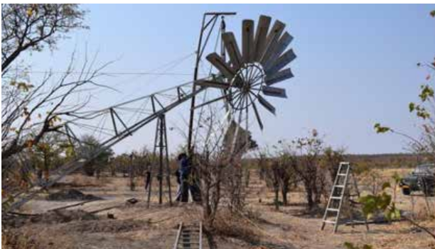
Installing a wind pump at Sinamatella pan.
