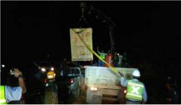
Loading transport crate into crane truck
