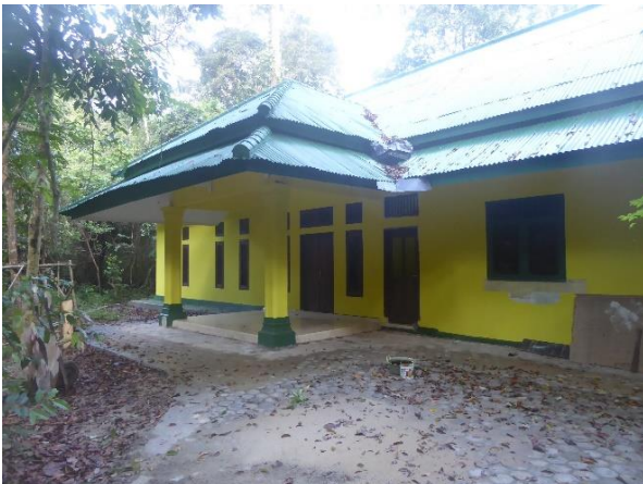
Figure 4: Exterior of the completed Laboratory. Credit: International Rhino Foundation.
