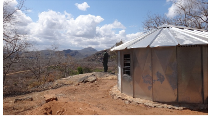
Figure 9. New security outpost. (Photo: GAWPT)
