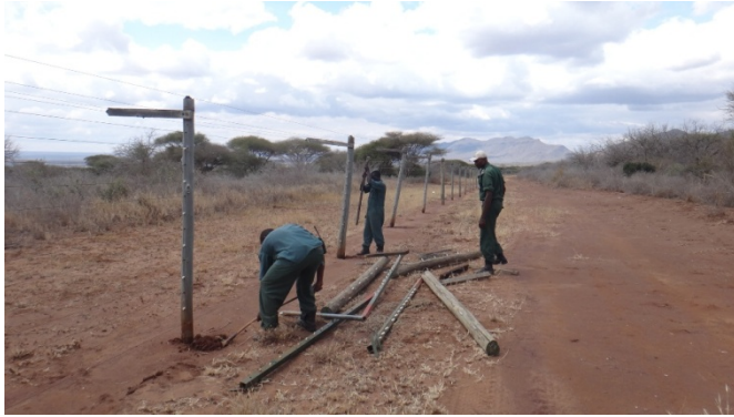
Figure 8. Fence construction. (Photo: GAWPT)
