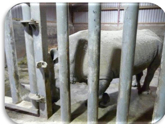
Figure 9. Strong steel door hinges
