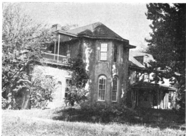
SPRINGDALE—THE HUFFNAGLE MANSION. Near New Hope, Bucks County, Pennsylvania. View from the west.
