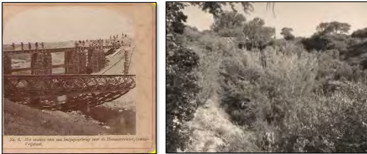
Figure 2.4: A stereo view image on the left (with no trees and shrubs) reading: “The construction of an improvised bridge over the Rhenoster River, Orange Free State.” Picture right, the same site, 117 years later.
