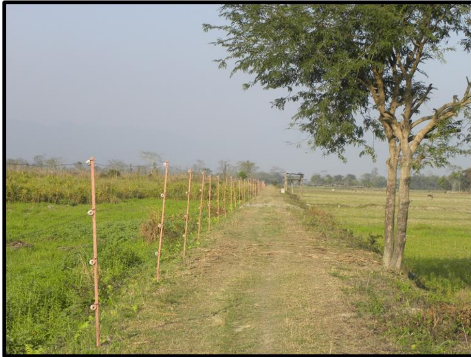
Photograph 5.17 Solar Electric Fence Erected at Southern Boundary of Manas to Prevent Rhino Stray
