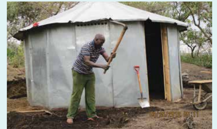
Works on uni-huts.
