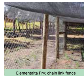
Elementaita Pry: chain link fence
