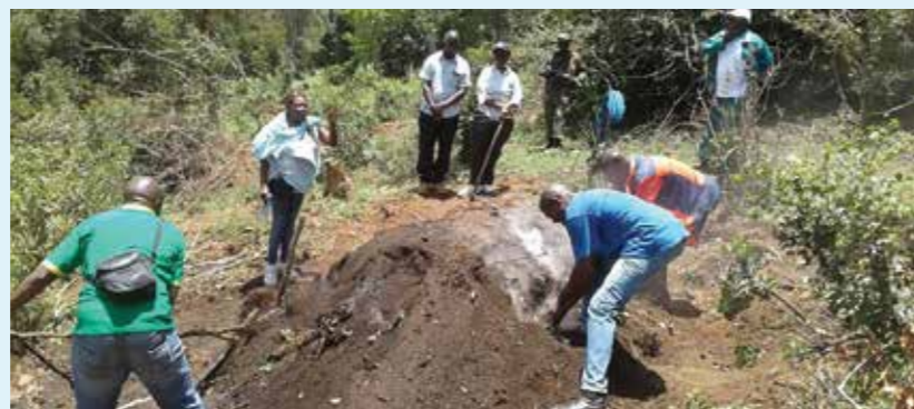
Landowners spearhead demolition of illegal charcoal kiln.
