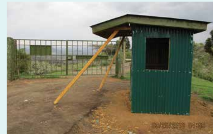
Gate shed under construction.
