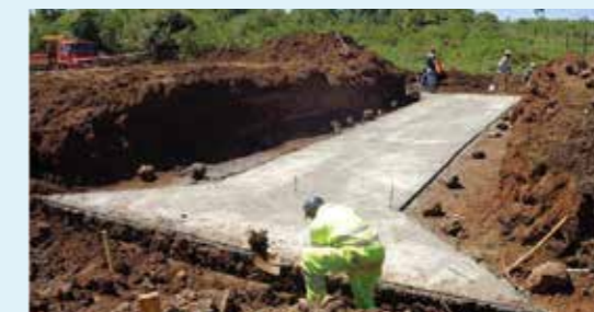
Animal Grid at Maili Kumi, Imenti Mt. Kenya Under construction.
