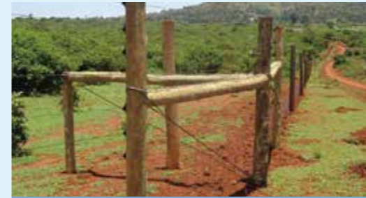
Outriggers added onto Rhino Ark Comprehensive Fence to deter habitual fence breaking elephants at Imenti, Mt. Kenya.
