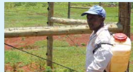
A farmer from the fence-line community admires newly built fence at Imenti.
