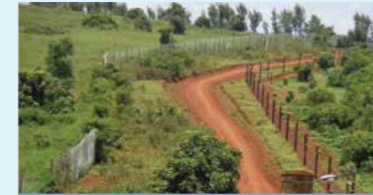
Progress on Fence construction at Lower Imenti opposite Meru University.
