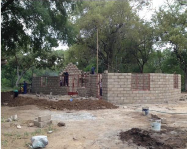
SSPU Manager's house and offices under construction
