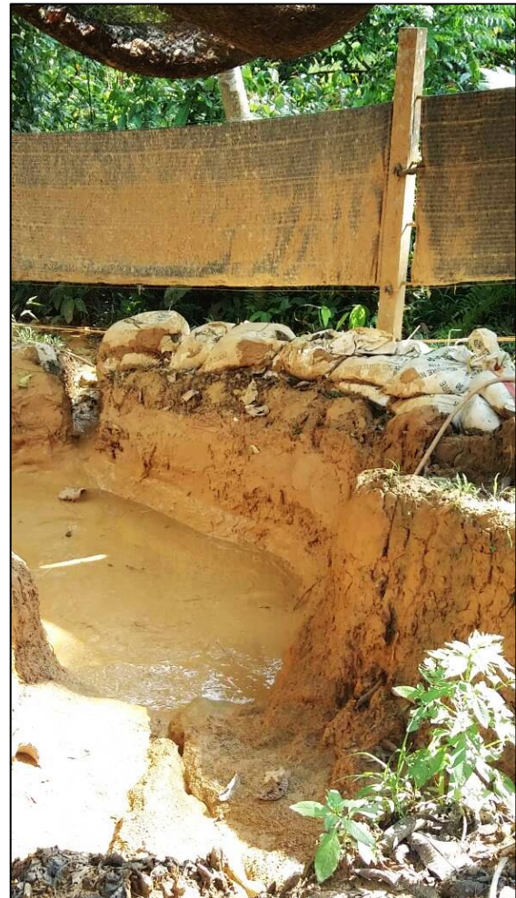
Plate 1. The sand bags were placed next to the fence to prevent Iman from expanding further
