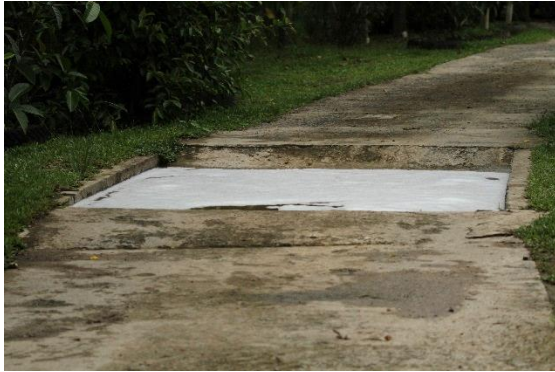
Plate 13. The two tyre bath (RIF and RQF) are constantly checked to ensure adequate disinfectant concentration is maintained at all times
