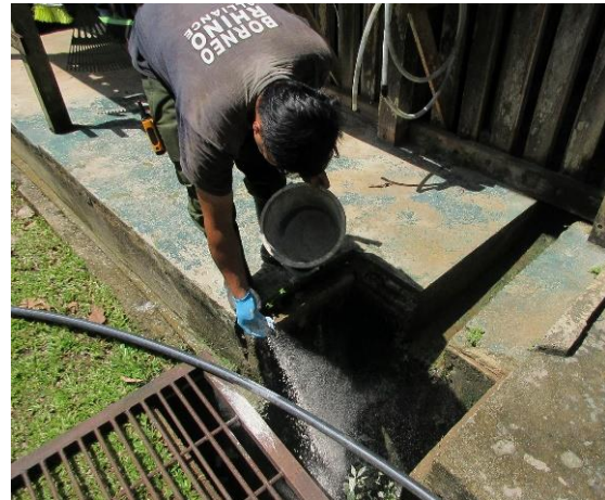
Plate 11. Wilson spreading lime into the sump at RIF
