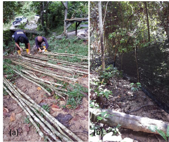
Plate 2. (a) Preparing the wooden posts and (b) the erected black shade net
