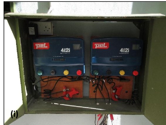
Plate 24 (g). The trees growing in the gutter of the staff quarters, (h). Plywood containers left under the water tank and (i) the two powerful energizers (16 joules), each able to power 120km of hot wire
