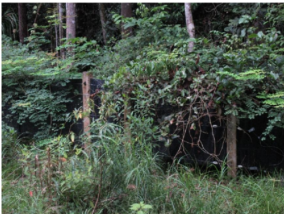
Plate 29. The fence almost covered by shrubs and creepers which can damage fence lines
