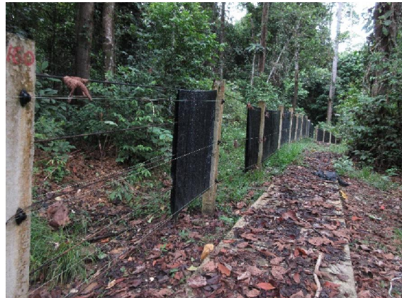
Plate 25. The black shade netting removed by elephants. The open fence lines encouraged wild pigs to move into the paddock
