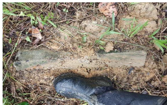
Plate 17. A part of the concrete posts partly embedded in the ground inside the paddock. The sharp hard edges are potential to the rhinos
