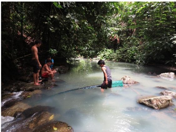
Plate 25. The repair at the gravity water intake
