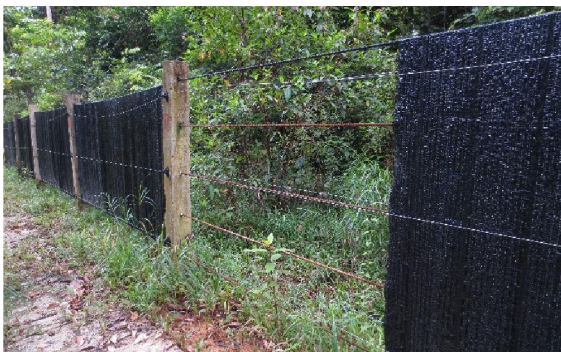
Plate 27h. The low or zero voltage on the fence need to be rectified as the capacity of the energizers is more than adequate to power the entire six fence lines.
