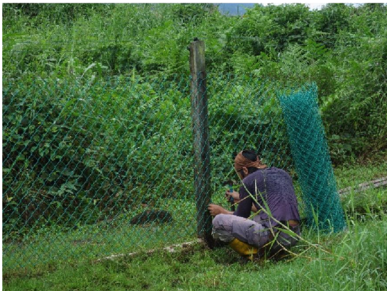
Plate 18. Davidson replacing old fence with new ones
