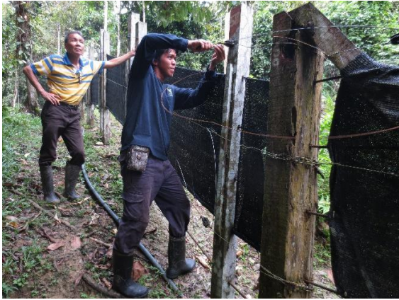
Plate 24. Samat Gubin replacing the rusty electric fence wires in RIF
