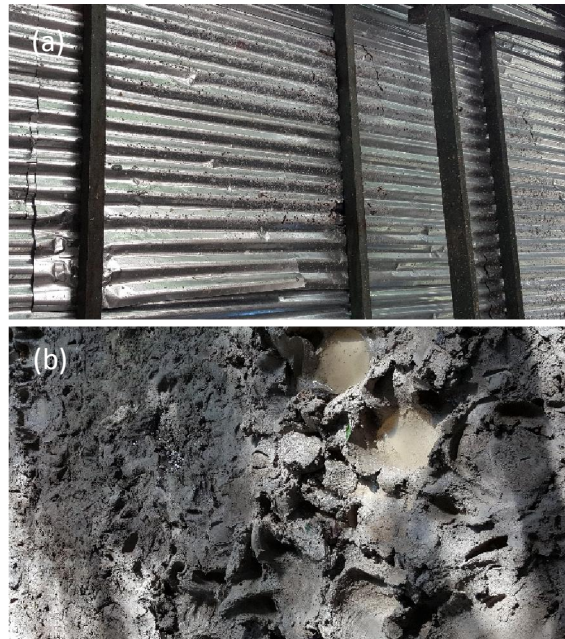
Plate 23. The poor quality zinc sheets with numerous holes (a) and (b), the puddles in her night stall
