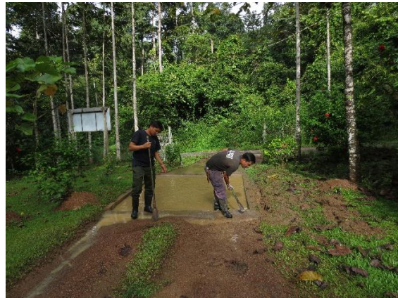
Plate 23. James and Wilson digging the earth drain
