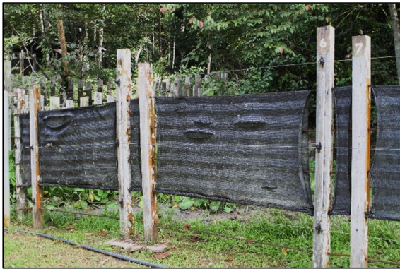
Plate 15. The torn black shade netting at RIF that affected some parts of the fence
