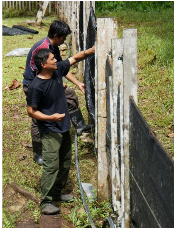
Plate 16. Wilson and Samat replacing the torn black shade netting from the fence in RIF
