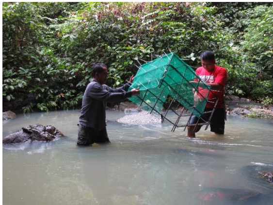
Plate 2. Replacing the filter at the water intake point
