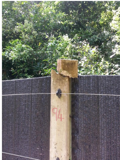
Plate 24. Broken top of the electric fence post.
