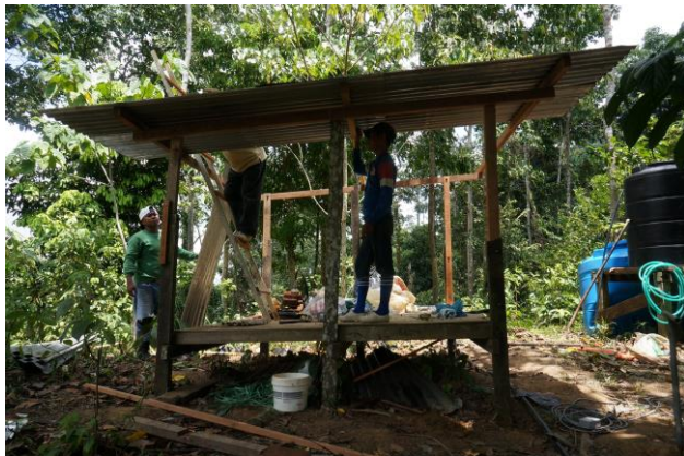
Repair and built new sheds in Rhino Food Plantation
