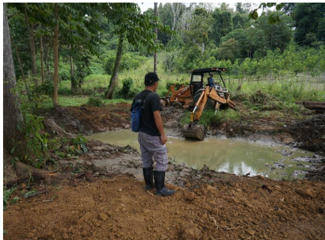
Enlarging the pond inside the plantation as water source
