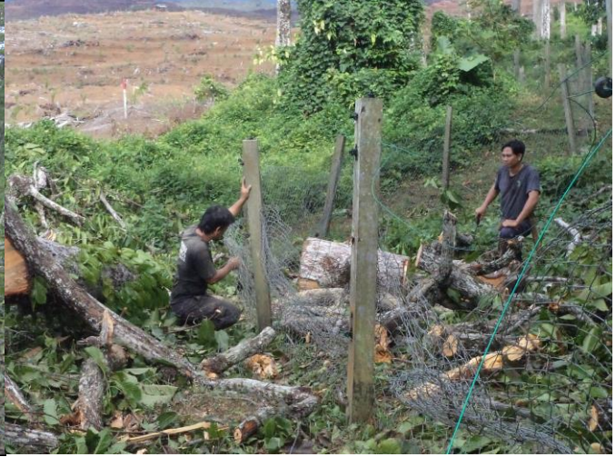
Repairs of fence by BORA staff
