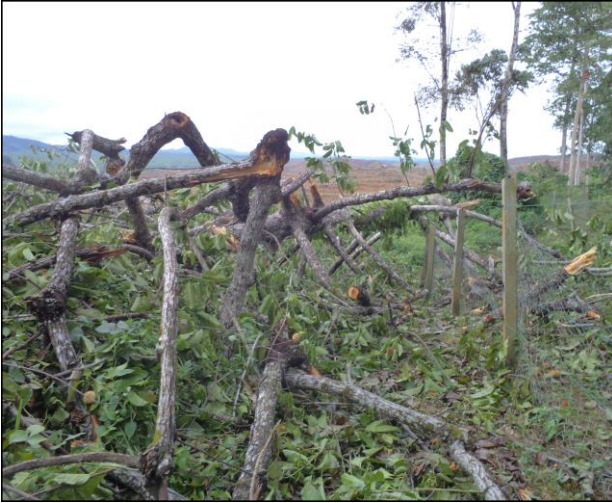
Fence damaged by tree fall
