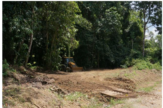
Repair of disposal site for rhino waste
