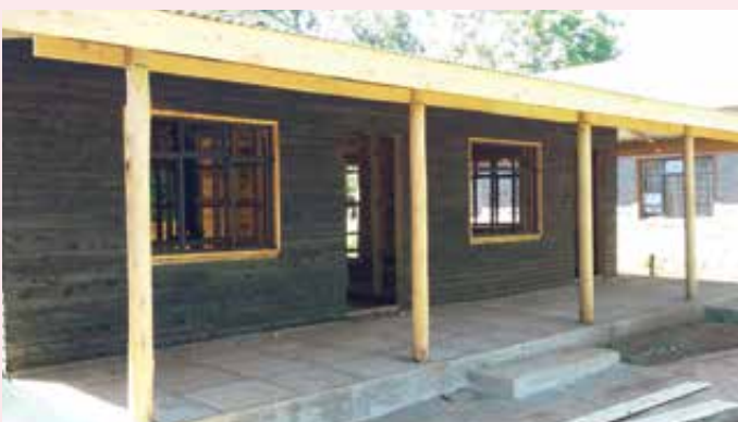
New Rhino Ark Nyeri Office under construction.
