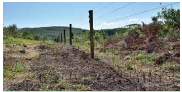
Completed and powered section of western boundary corridor fence
