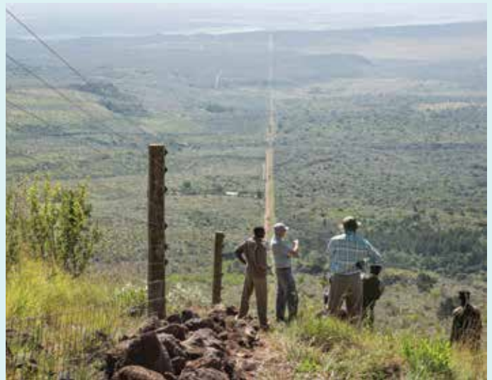
Completed fence facing Lake Naivasha
