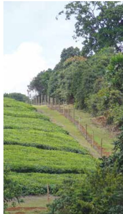
Electric fence, Phase I (Kiringa River – Thuchi River)
