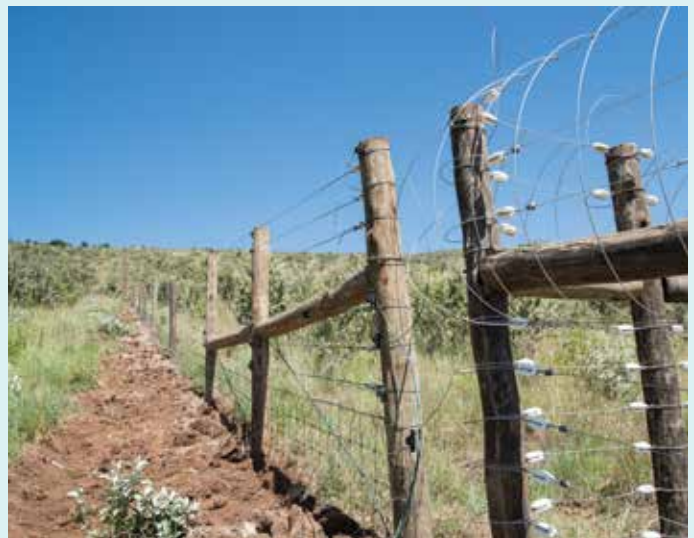
Meeting point between completed Loldia Fence and Green Park Fence
