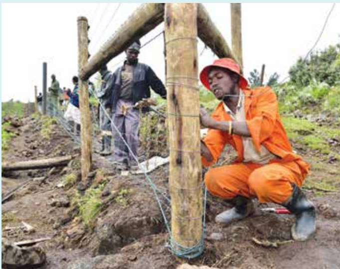
Fence construction work
