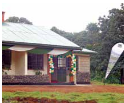
Completed energizer house at Castle Forest Station (Phase I)
