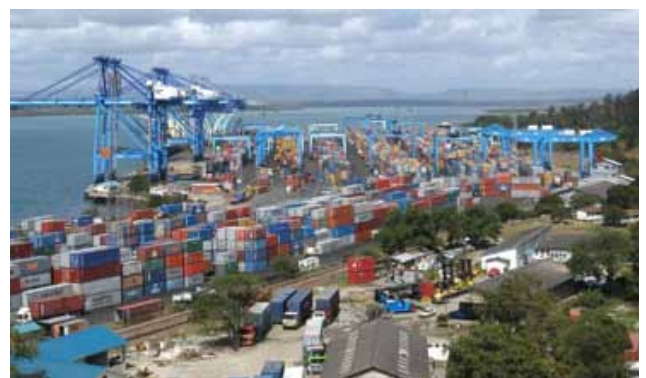
2013, container hub in Mombasa harbor
