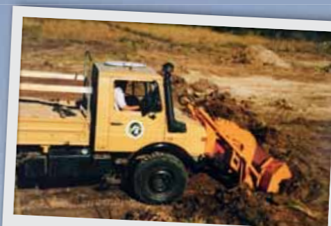
Work begins on the North Luangwa airstrip.
