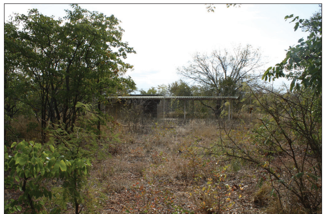
Figure 5 Masokosapan's jail surrounded by a still-intact razor-wire fence (photo by author 2009)
