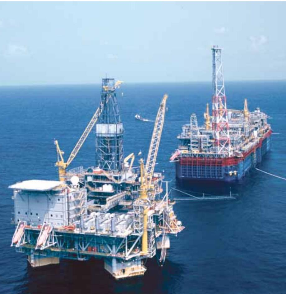
Sanha platform gas compression totals 198,000hp. This one project will eliminate around 41 per cent of Block 0 gas flaring compared with 2003 flared volumes.
