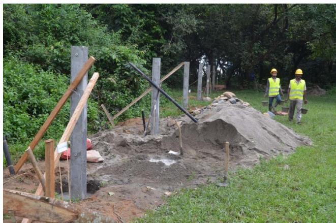
Figure 8. Fence construction in UKNP
