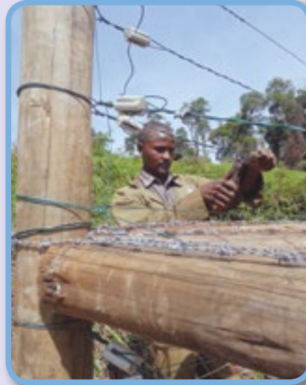
Strainer assembly under construction near Chuka Forest Station
