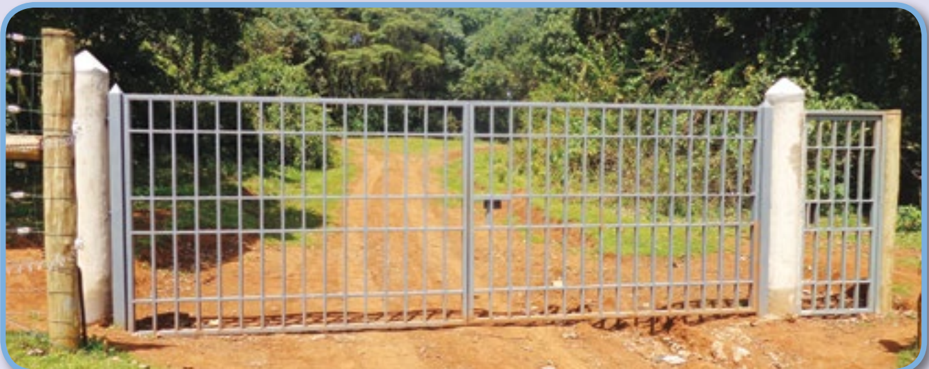
Newly built gate along Mt. Kenya Electric Fence
