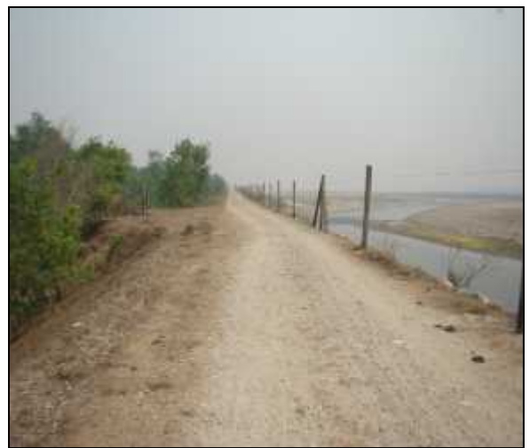
(xii) Electric fencing to restrict rhinoceros movement along Rapti River bank.
