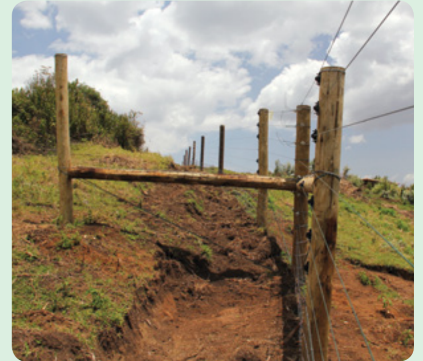
Corner strainer assembly at completed section of fence in Gachuma area
