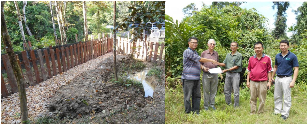
(left) pebble walkway constructed to allow Puntung to more easily walk up and down the slope (compare with same site shown in previous quarterly report), (right) agreement to commence construction of the BRS Danum facility (30 October) pending re-alignment of the facility further from the roadside (left to right in picture : Mr Wong (Buildtech), J Payne (BORA), Indra Sunjoto (District Forest Officer; DFO), Jikos Gidiman (Danum Valley manager), Robert Mijol (Assistant DFO)
