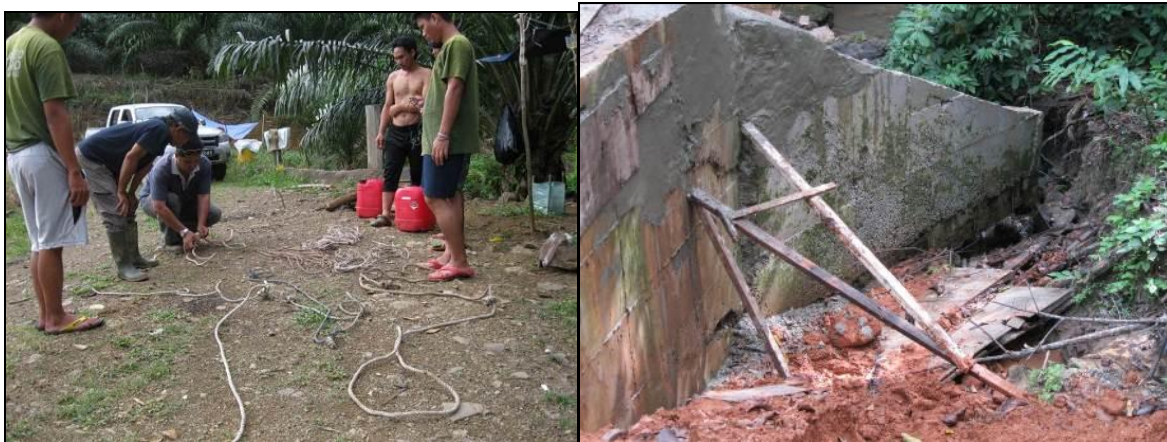
(left) 10 jerat (snare) ropes retrieved from forest near to the Kulamba rhino trap (February 2012), three are big enough to cause the death of a rhino, (right) view of the BRS access road ("Pakej A") box culvert (6 June), showing additional "patching up"
