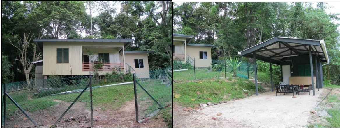
(left) BORA field manager / veterinarian's house and (right) garage were renovated in June
