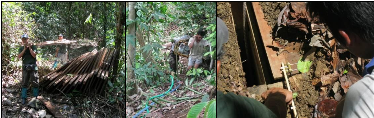
(left) materials for trap 5 (about 6 km from forest edge), including a temporary stockade for use after capture, were brought in to the site by manpower over a period of two weeks, (middle) a water pump and piping is installed to obtain water from a small stream 150 metres from trap 5, (right) an electronic device was installed at trap 5 in an effort to be able to monitor the trap without twice-daily manual checking.
