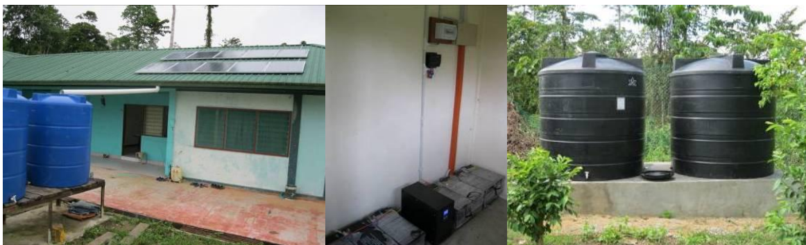
(left) the ten photovoltaic cells for solar electricity at RQF were installed in mid November, (middle) the electrical storage batteries, (right) the piped water supply to RQF remained unconnected by end of this quarter, and the two new water storage tanks at the RQF had to be filled manually.
