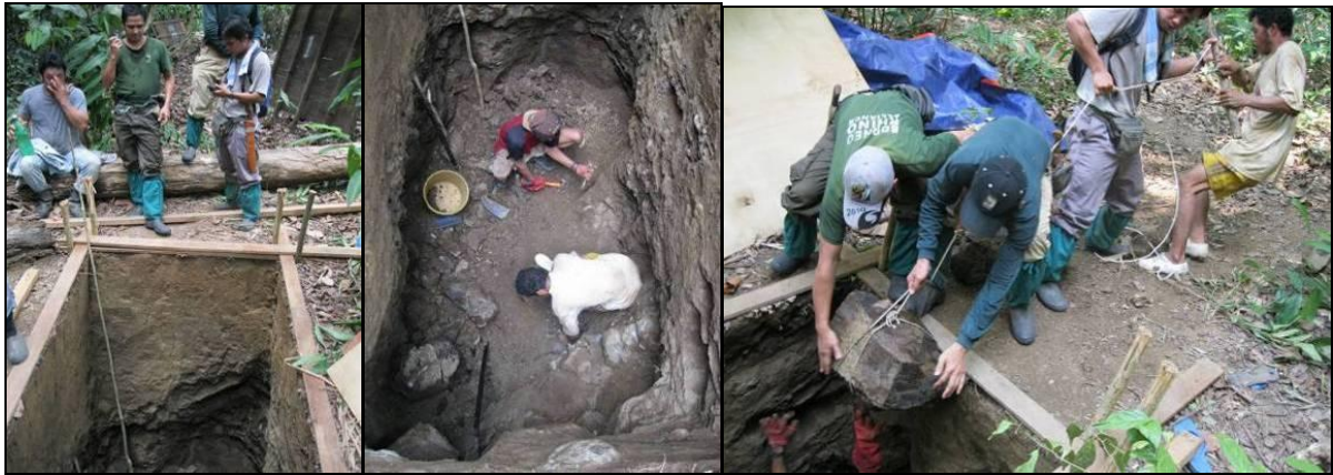
(left) digging the hole for trap 5, (middle) a view inside trap 5 hole during construction, the rock is removed by chisel and pick axe down to a depth of eight feet, (right) removal of rocks from the trap 5 hole during construction.
