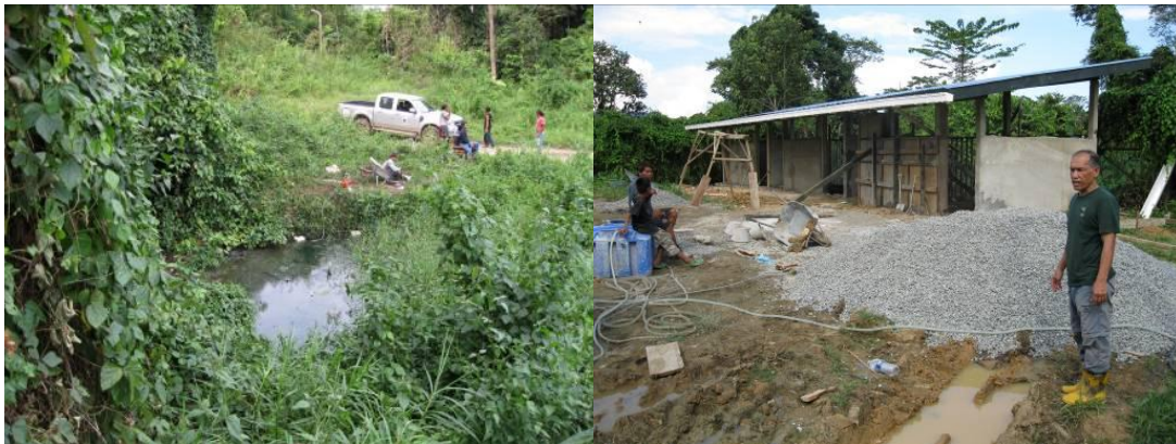
(left) a spring (“mata air”) exists within 80 metres of the Rhino Quarantine Facility, but it was found to dry out during non-rainy periods, and being near the public roadside there is a risk of pollution, so is unsuitable as a water source, (right) construction of the RQF underway in late June.
