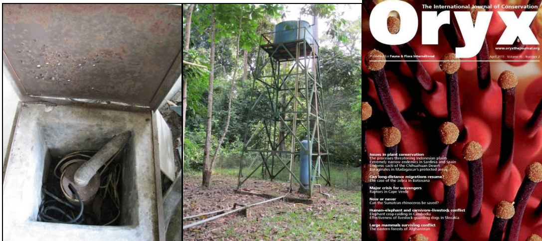
Sumatran Rhino Sanctuary (SRS) at Way Kambas : (Figure 17, left) view from the top of the 100 metre deep borehole and sole water source since 1997, (Figure 18, middle) the raised tank which supplies water to the staff and visitor buildings, and to the rhino paddocks via about 4 km of pipe. (Figure 19, right) April 2011 edition of Oryx, which contains a “Now or never” paper on the Sumatran rhinoceros, highlighting Borneo Rhino Sanctuary.
