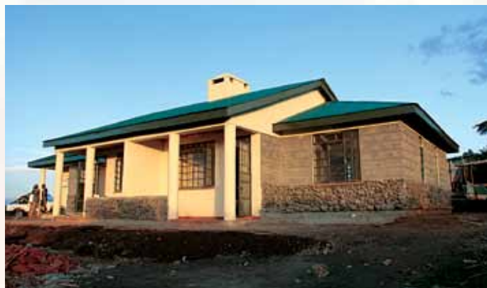
Morop fence energizer station
