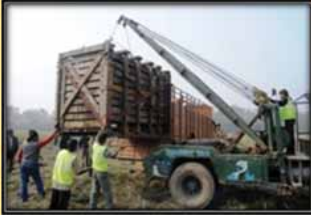
Loading crate on to truck
