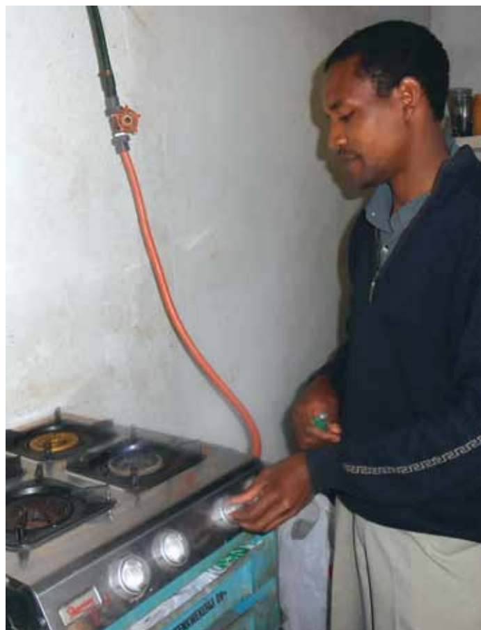
Gas from the units is piped to a conventional domestic gas burner
