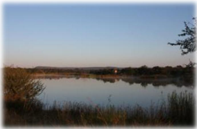
Permanent dam constructed in stream
