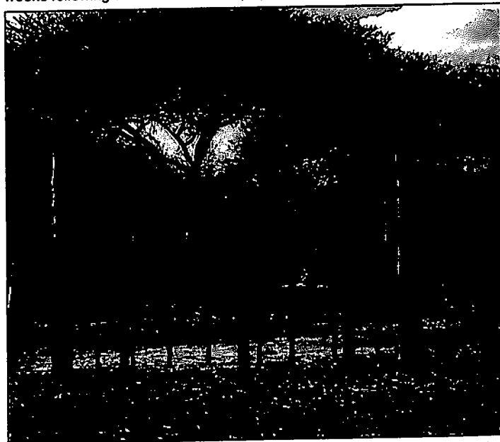
The fencing of the natural enclosure was visually highlighted using added poles shorter than the main poles plus adhesive tapes. (dh)
