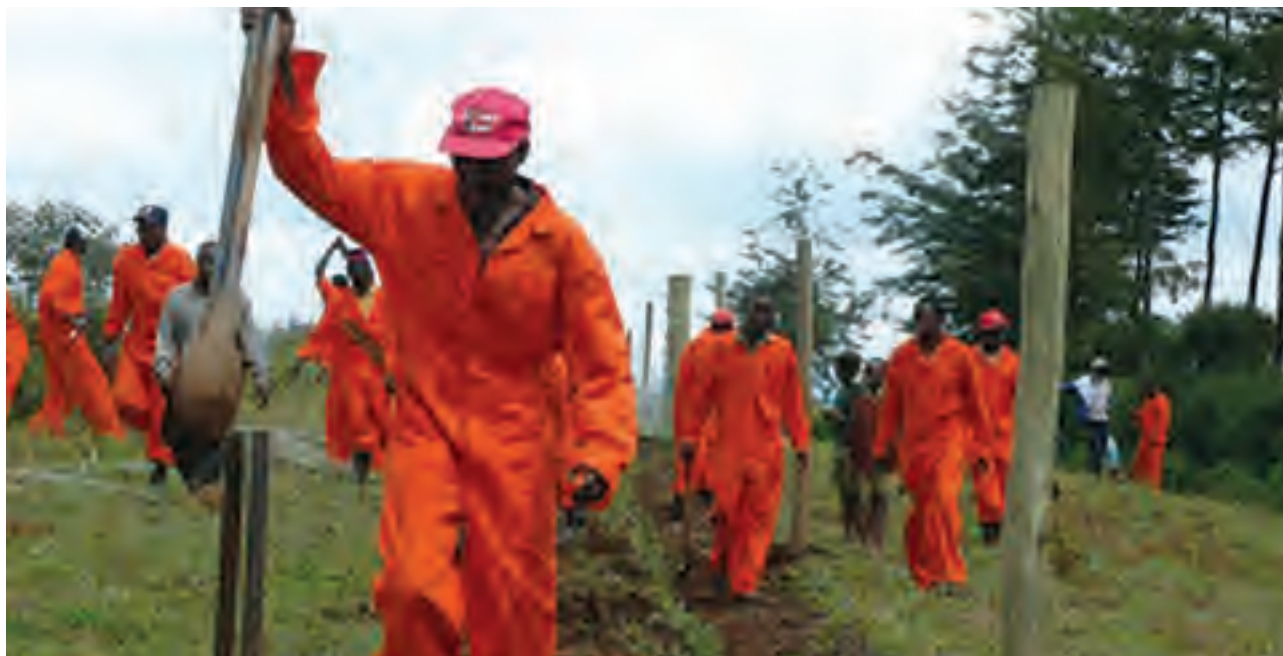
Fence construction work
